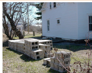
2. Cement blocks are cleaned and stacked ready to use
