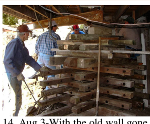
14. Aug 3-With the old wall gone, the house rests cribbing supporting the steel beam brace
