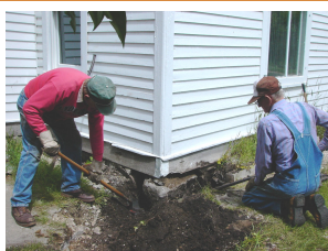
10. Aug 1-Preparing for the jacking, Pete Anderson & Herbert Ongstad remove large stone from SW corner
