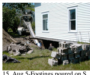
15. Aug 5-Footings poured on S and SW portions with help of Paul, Wanda, and Herbert
