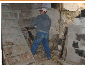
18. Aug 15-Jacob removes a coal bin partition, in preparation for third phase of wall work to come
