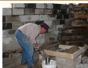
19. Aug 15-Pete 'butters' the ends of the cement blocks with mortar
