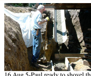
16. Aug 5-Paul ready to shovel the cement along the channel of the footings frame
