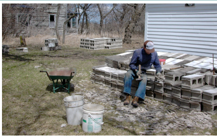
Herbert Ongstad using a chisel and hammer to loosen old mortar from cement blocks.
