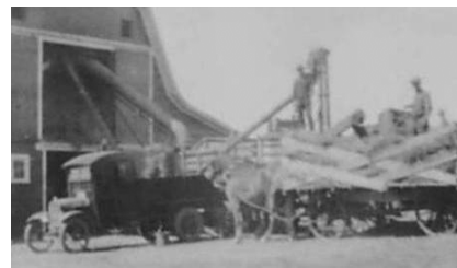
The straw blown directly into the barn from the separator, and the grain is collecting in the 1928 Chevrolet truck.
