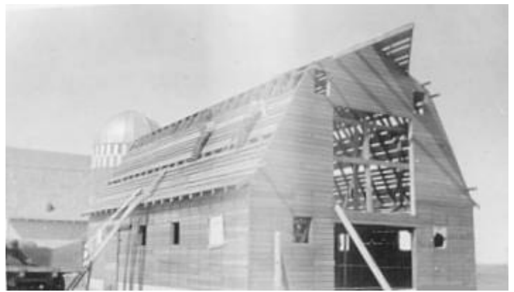
The construction of Ben's second barn in 1945. Ben and the hired man Willis Westman are shown on the roof, nailing roof boards in place. The barn built in 1941, appears in the background.
