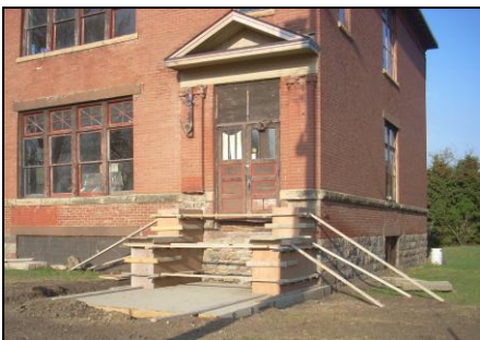
4 Second pouring – side platforms curing
