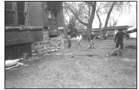
3 First pouring – finishing the base
