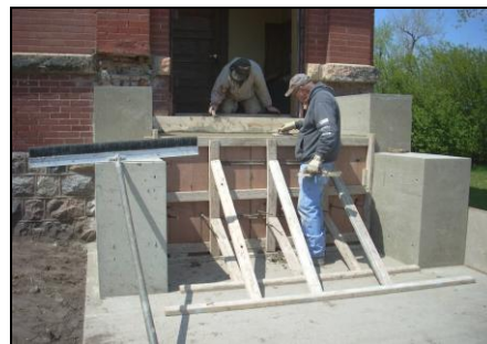
5 Third pouring – top step and landing
