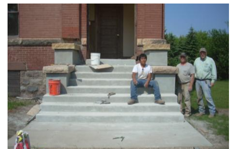
9 Installation of cap stones completed
